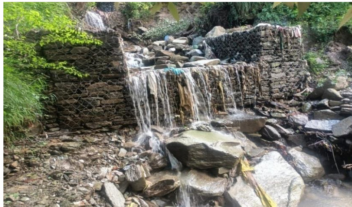
Figure 14.2 Stony Check Dam
